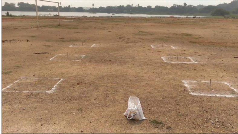
MARKING OF FOUNDATION
